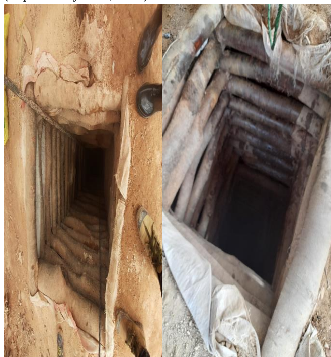
Plate 1: Pits constructed using Brachystegia spiciformis (left) and Eucaryptus paniculata (right).
