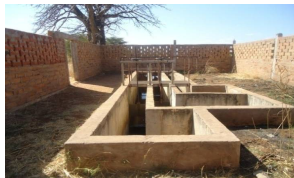
Plate 4: Water distribution chambers for irrigation canals in Hombolo (Photo by: Author, August 2016)
